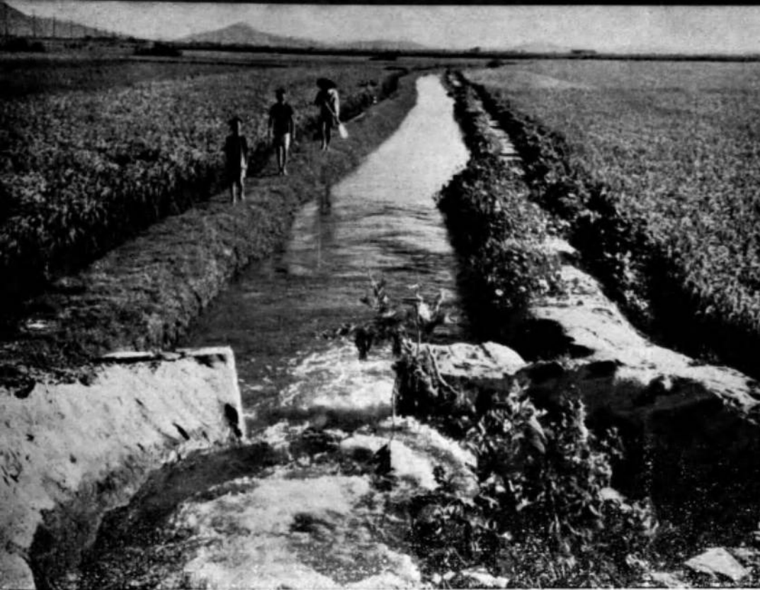
A new irrigation channel in the outskirts of Wusih, Kiangsu province. Water is supplied by power-driven pumps.
